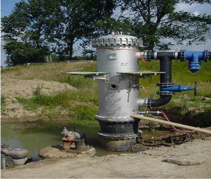
Figur 26: Lance installation for pigs in a pressurised pipe [10]
