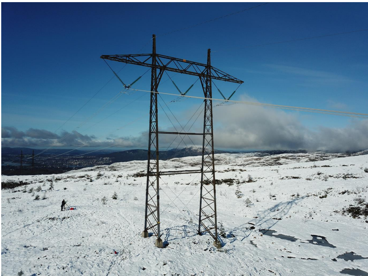
Figure 3 Electricity pylon at test site (own image)
