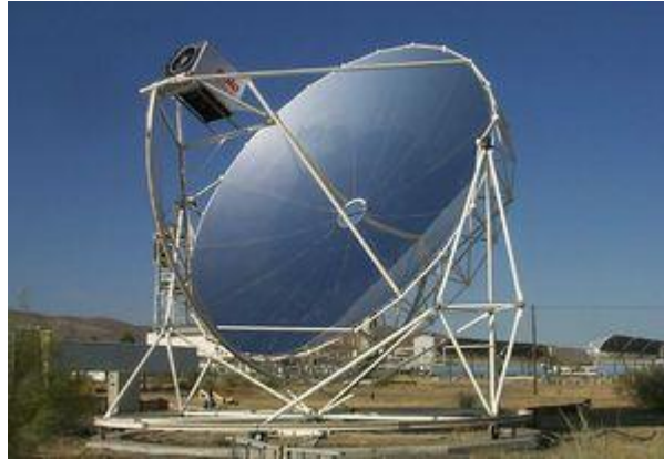
Figure 10. Parabolic mirror with a Stirling engine on its focus
