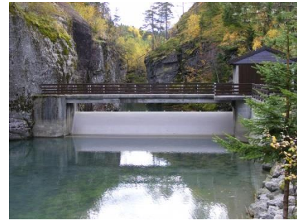
Fig. 6 Dam at outlet Veitstrandvatnet
