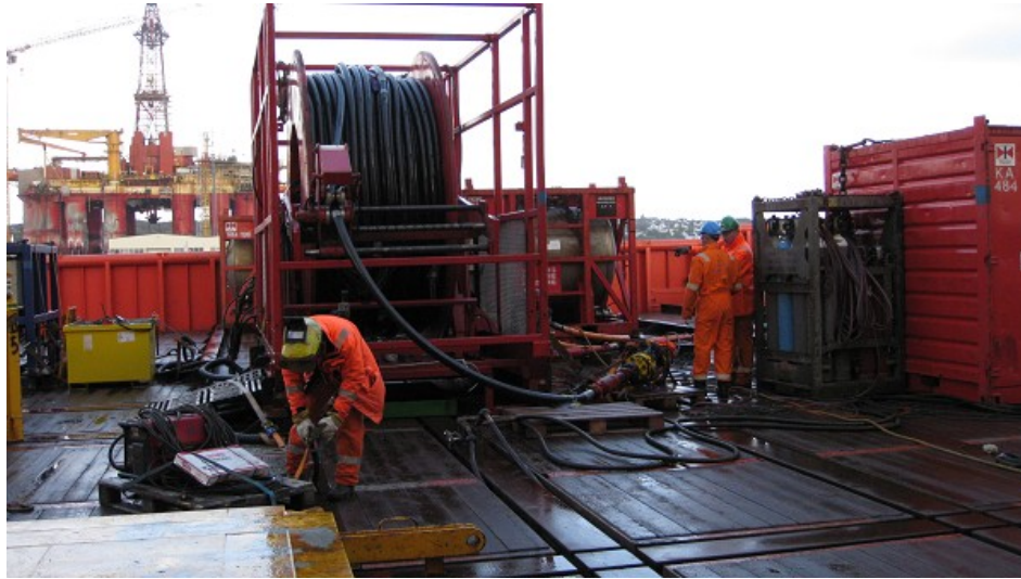
Photo 2: Cargo being welded to the main deck during mobilization
