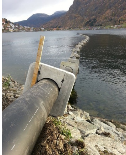
Figure 1. This picture was taken during the construction period and shows the hose before it was filled with sea water and sunk to the seabed. For stabilizing purposes, weights made of concrete were attached to the hose. This picture is from a WEPS built in the municipality of Sogndal in 2014 by Sognekraft AS. The picture is used with permission from Sognekraft AS, Norway.
