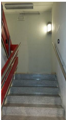
Figure 5: Intervention site stairs
