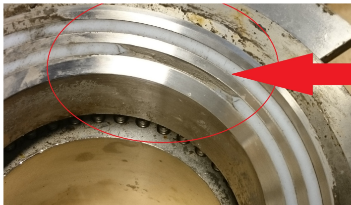
Figure 2.1: The damaged gasket
